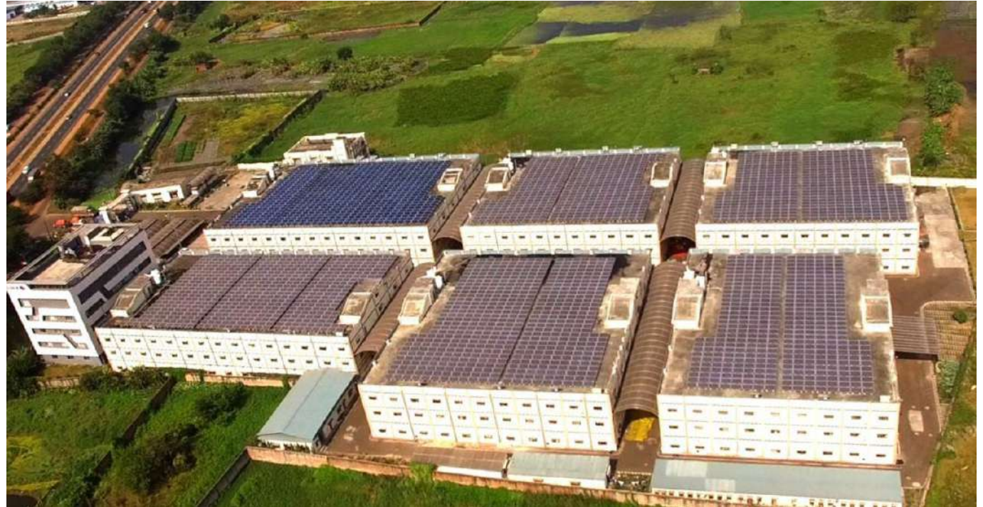
Rooftop solar power plant at Dankuni unit
