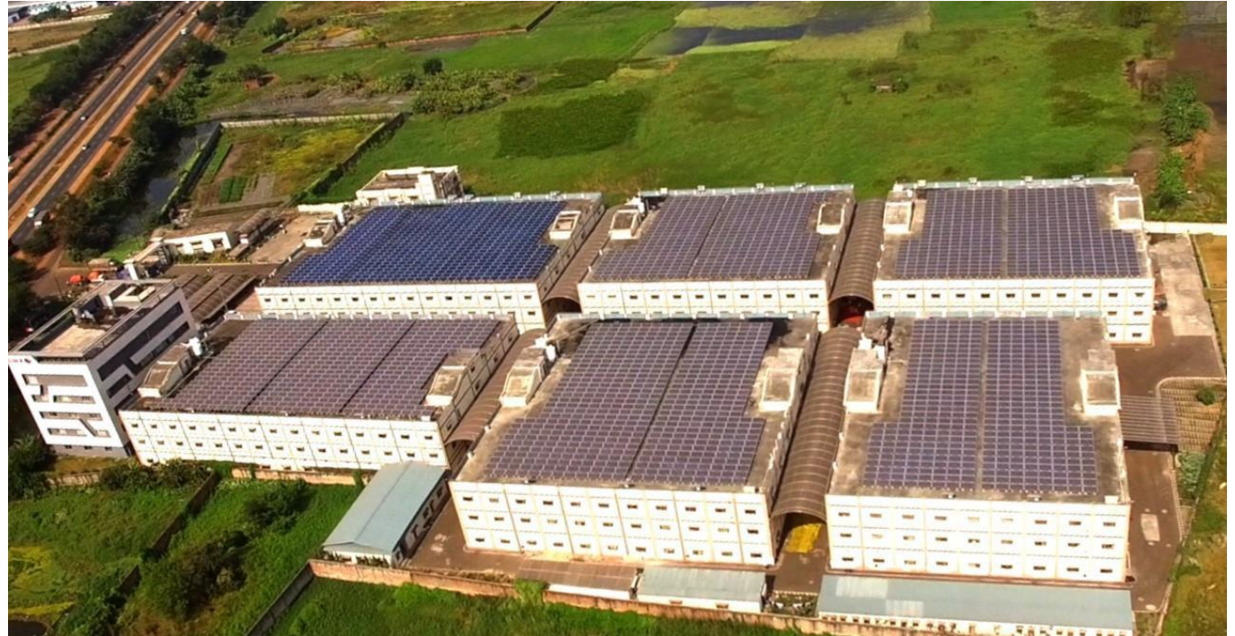
Rooftop solar power plant at Dankuni unit
